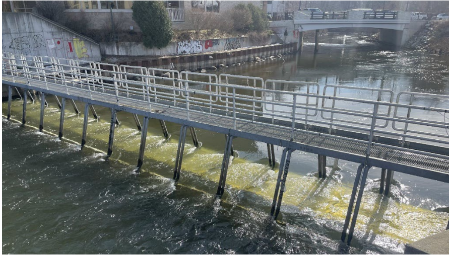
Figure 3. Horizontal submerged screen weir (HSSW) installed at the MI DNR Traverse City Salmon Weir on 18 March 2025. The HSSW is designed to capture a portion of sea lamprey migrating along the bottom of the river while allowing other fish to swim past. If successful, the HSSW could help researchers assess sorting technologies at FishPass.
