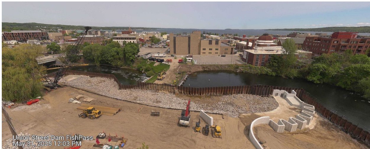
Figure 1. Image capture from the FishPass time-lapse camera: May 31, 2025 showing the nearly complete arc-labyrinth weir (right side of image) and temporary bypass channel. Water flows from right to left.
